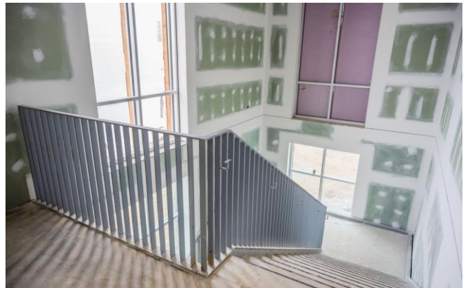
Stairwell ready for paint 12/07/2022
