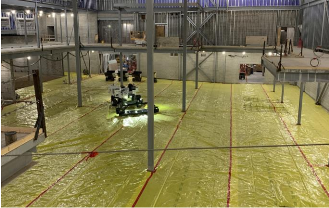
Cafeteria floor prepped and ready for concrete 12/07/2022
