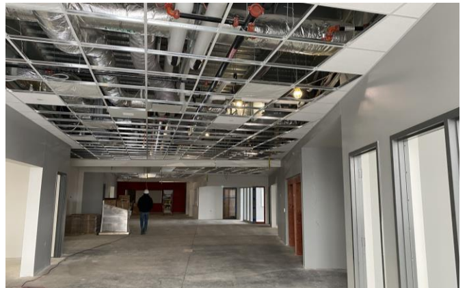
Ceiling grid in hallway outside of classrooms 12/21/2022
