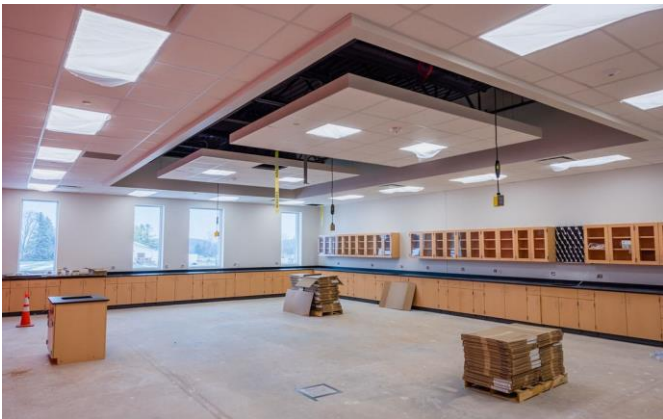
Completed science lab ready for flooring 12/07/2022
